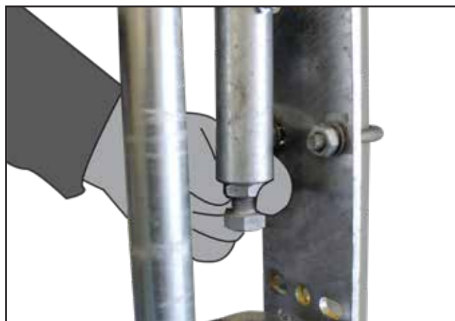
J. To tension the hinge loosen the locking nut as shown.
